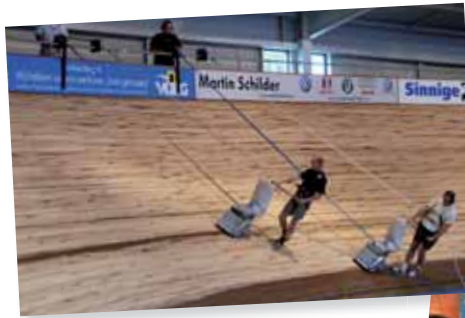
Bona Belt was used to sand the cycling track at Sportpalais in Alkmaar in the Netherlands with a slope of up to 42° on the curves.
