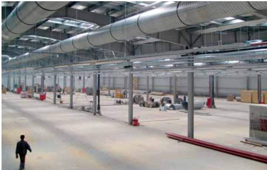
Work progresses on the new parquet factory in Kaluga
